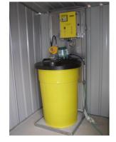
MCD 200 Series pH Controller / Monitor / Data Logger and Polyethylene Chemical Storage Tank fitted with Chemical Pump and Agitator.
